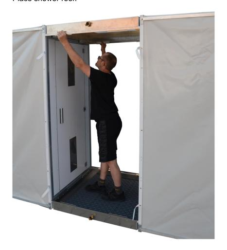
Ensure that the shower roof snaps behind the profile of the chambers.
