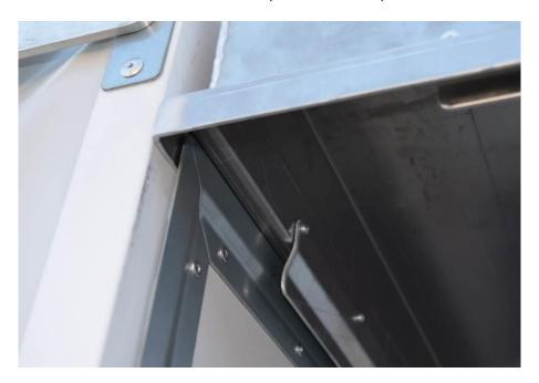
Insert wall elements of the shower chamber into the guides of the floor element and at the same time ensure that the corner profiles snap behind the guide profile of the chambers.
