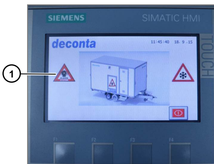
Fig. 1 67 Status of the alarm system
